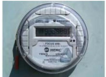
*AMI meters do not rely on gears and rotating disks. These meters are used exclusively throughout HEMC's system.*
