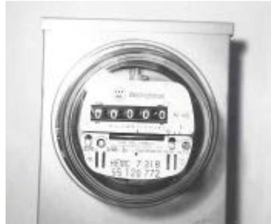
*The electromechanical meter uses intricate gears to accurately measure the amount of electricity used.*
