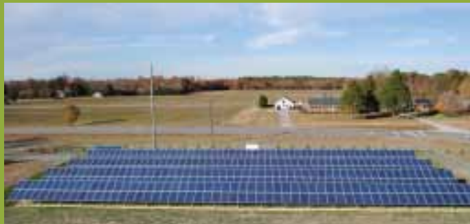
Bright Star1 Green Energy Plant
